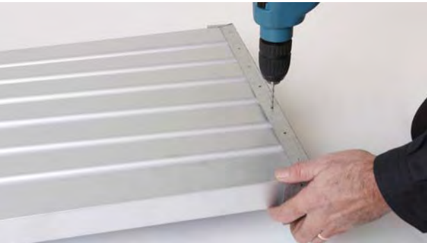
2. Drill rivet holes
